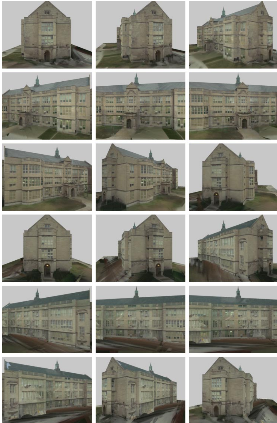
Figure 6.7: University High School fly-around, without trees. For this sequence, which is the same camera move as in Fig. 6.6, the trees were masked out of the twelve original photographs of the building using the technique of Section 6.5.2. The masked sections were then filled in automatically by the image composition algorithm.
